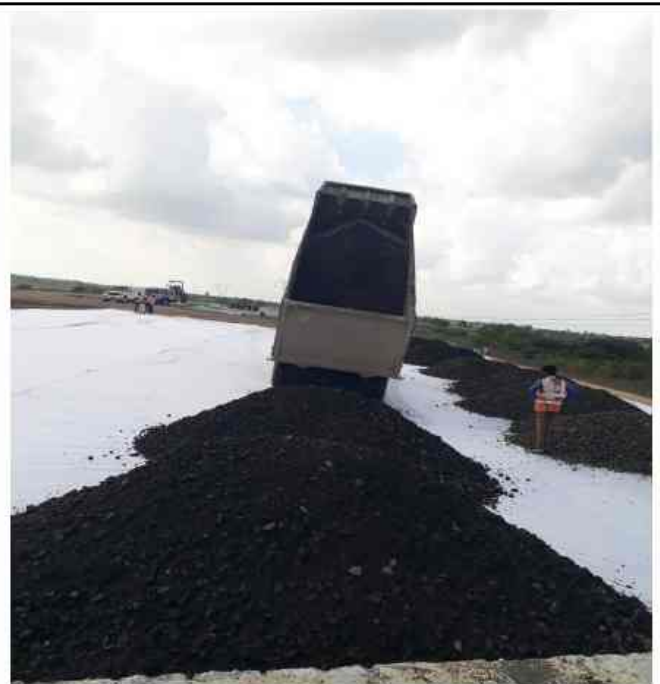
312+694 GSB dumping work in progress at A1 side.
