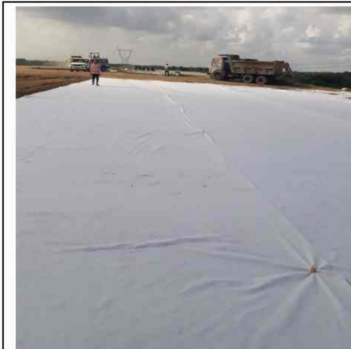
312+694 Geo textile laying at A1 side.
